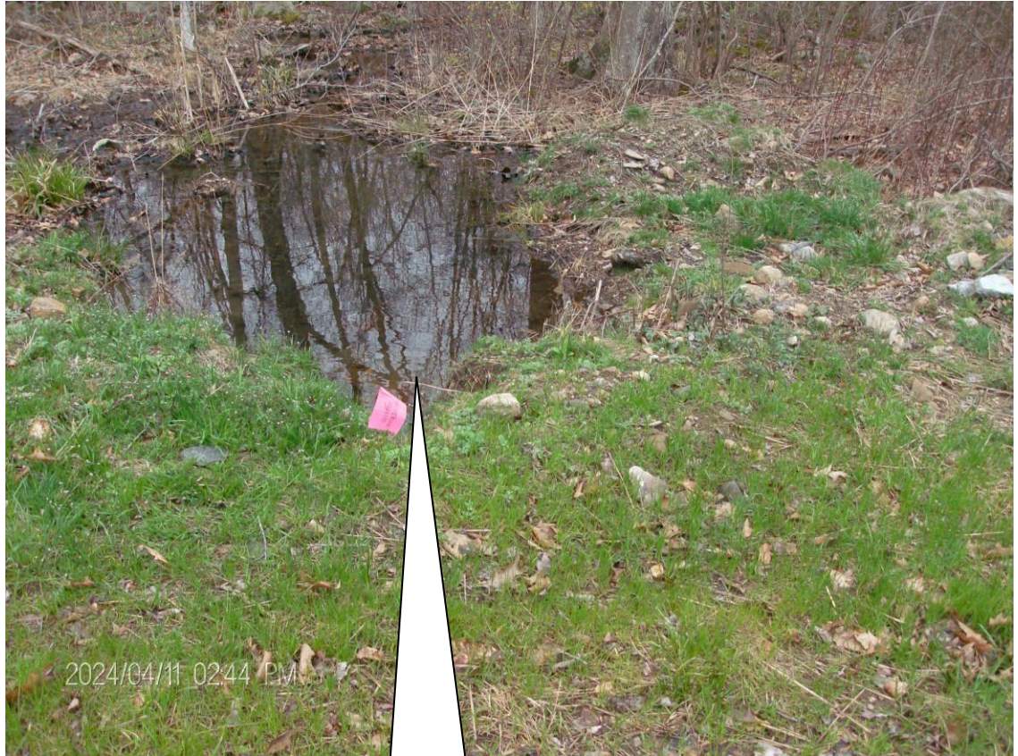
Culvert outlet location at edge of flagged wetlands
